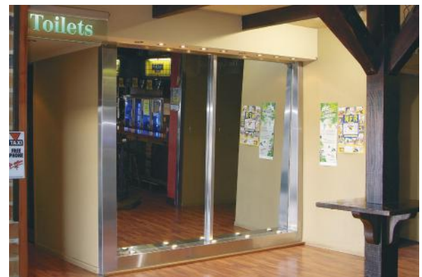
Laminated one way mirror – Subject side view from outside of men’s restroom, lighting maximised to prevent see through.
